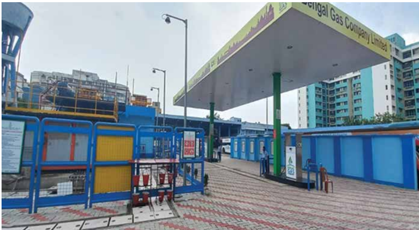
CNG Station at Kasba (COCO) , BGCL
